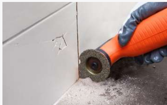
Routing joints right into 90 degree corners
