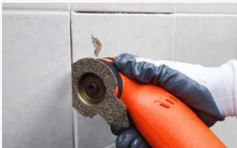
Routing joints on wall and floor tiles
